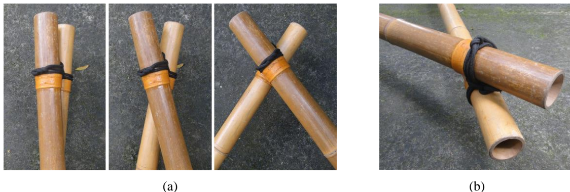
Figure 2: Hinged lashed connection (HLC). (a) HLC articulated mechanism. (b) Detail of HLC
